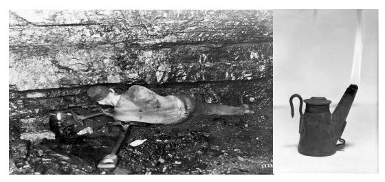
After the coal was shot down and the smoke had cleared, the miner's next job was to shovel the chunks of coal into little rail cars that would later be pulled out of the mine by mules or oxen [see picture below]. Needless to say, there was nothing about coal mining in 1876 that was either easy or safe, but the under-cutting operation was, far and away, the most time consuming and the most dangerous.
